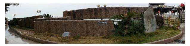
Fig. 4. Ancient granite stone beams of the Guangji bridge (number 12), preserved in a park near the bridge. The spans range between 10 and 14 m.
